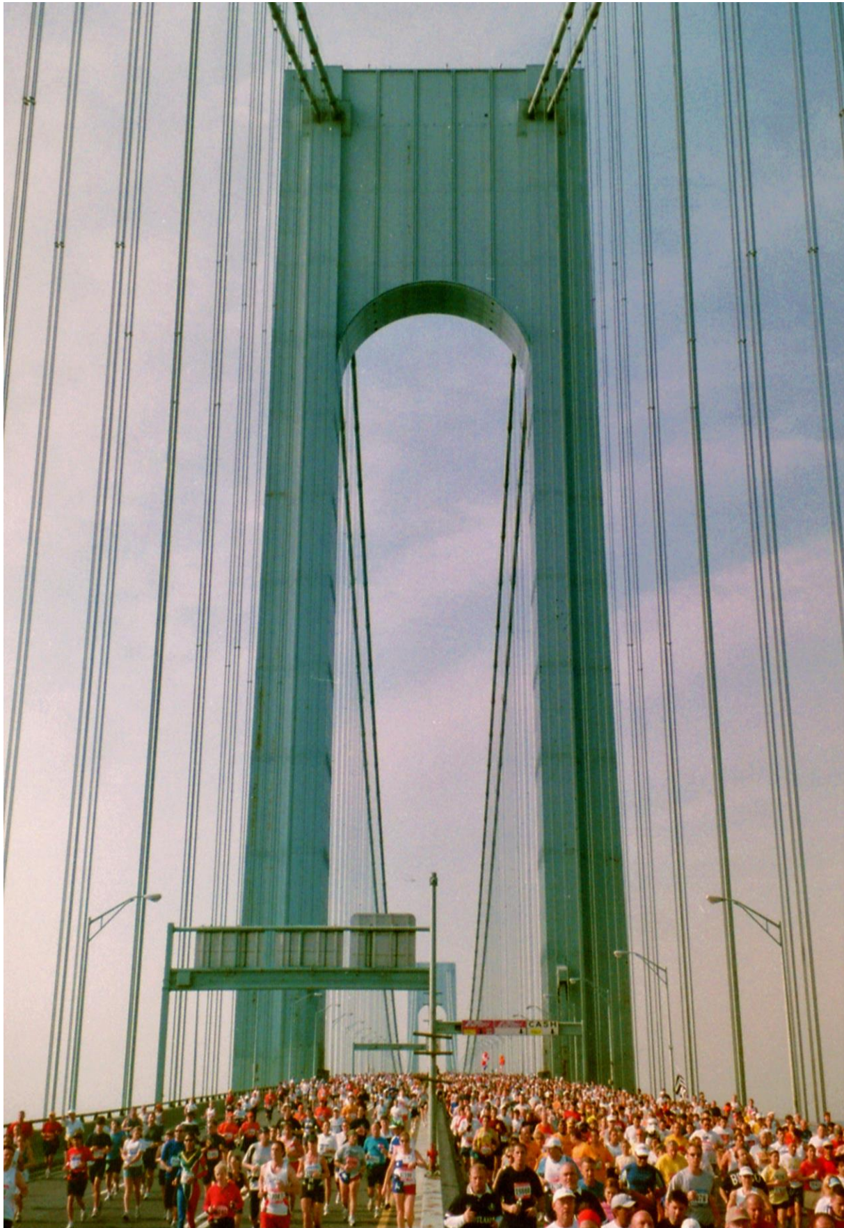
Verrazano Narrows Bridge
